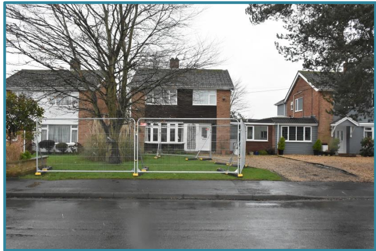
Figure 19. HERRIS fencing braced and secured with weighted boots
