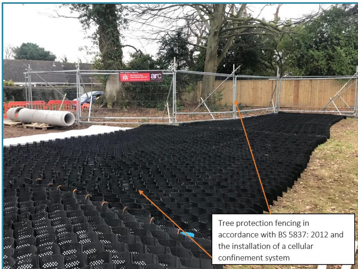
Figure 18. A 3D cellular confinement system, laid and secured with road pins and awaiting infill with washed angular stone to complete the ground protection and later to base the new driveway upon
