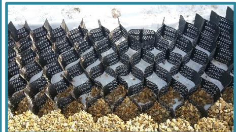
Figure 11. A cellular confinement system awaiting infill
