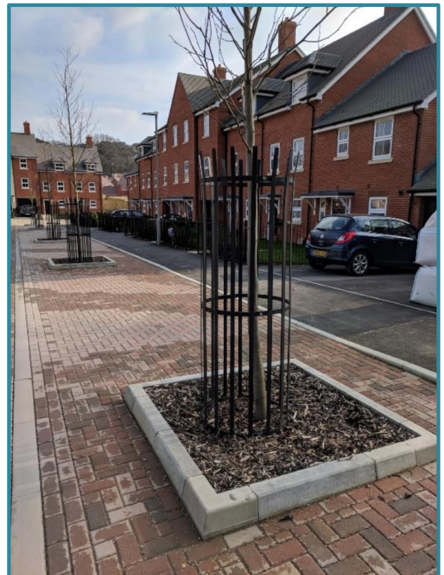
Figure 29. A newly planted avenue of street trees that have been successfully incorporated into the sites SUDS
