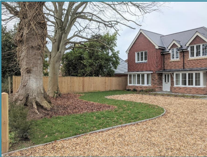
Figure 12. A new access and driveway situated in close proximity to protected, mature Oak and Beech trees through the use of a 3D cellular confinement-based surfacing system
