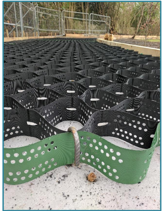
Figure 28. A cellular confinement-based driveway, awaiting infill with washed stone
